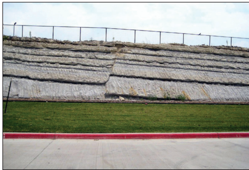
Figure 8. Highway outcrop of Cretaceous Austin Chalk, Dallas County. Note normal fault in the center of the photo.
